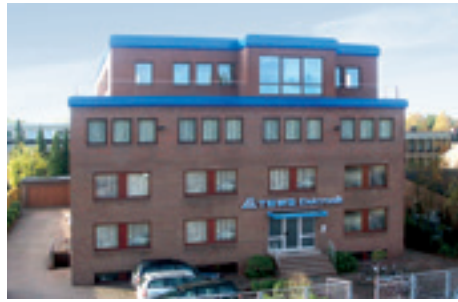
Another storey added to TEWS Elektronik building in Hamburg, summer 2005
